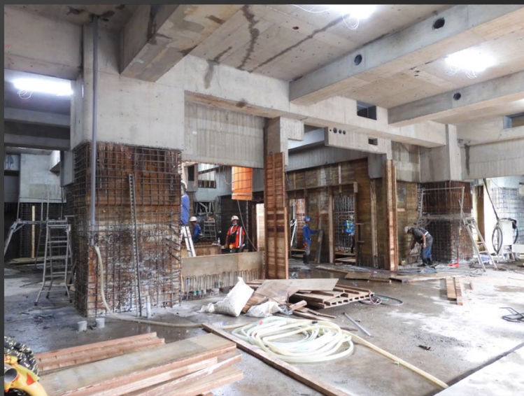
H棟B1F柱牆結構體施工 2021. 10. 12
