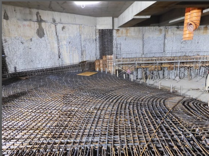
G棟B1F北區車道結構體施工 2021.11.19
