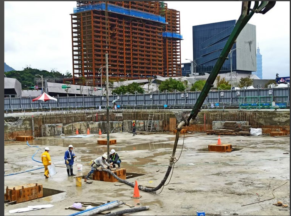
柱內無積水確認.柱內灌漿
