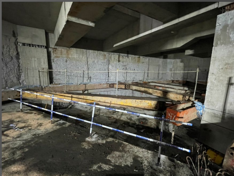
G棟B1F北側車道水平支撐 2021.12.27
